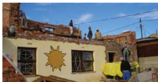
A new home in the making!
